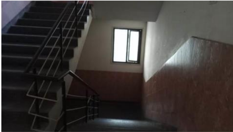
Staircase receiving daylight through windows
