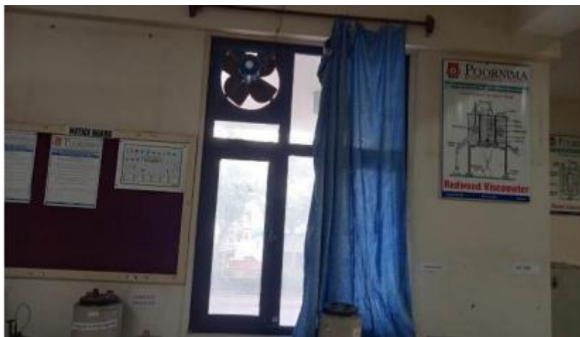
Exhaust fans in labs
