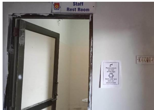
Water conservation Signage in Restrooms
